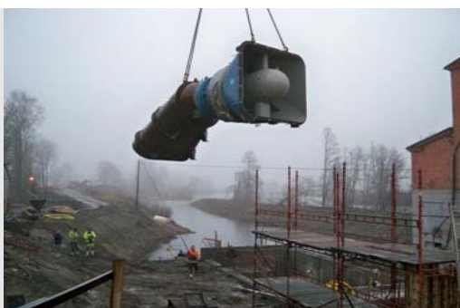
The Kaplan S bulb turbine is inserted
