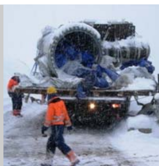
Delivery and assembly of the two Francis spiral turbines
