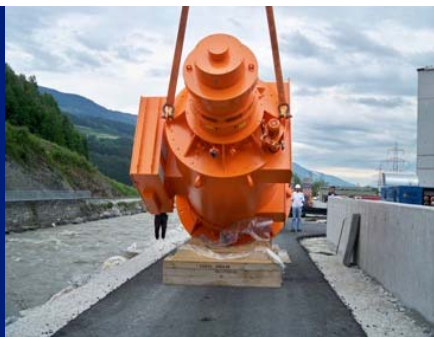
Assembly of the turbine and the 33 ton-generator
