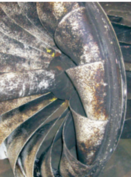
Francis runner before modernization.
